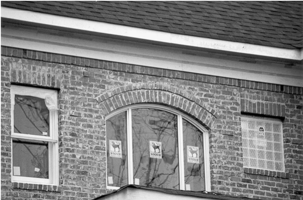
Notice the substantial reveal between the brick trim and the main body of the home. This should be a minimum of \frac{3}{4} ".
